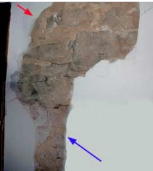
Red Arrow shows mortar with exterior finish. Blue arrow shows rough, unfinished interior garret mortar. Pencil diagonal line drawn on plaster shows the conjectured south roof slope, based on mortar.
