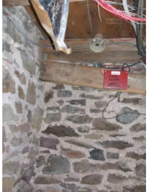
Current floor joist above old, sagging floor joist along east end of "B0" cellar. North end of old joist embedded in "B0" fireplace mound.
