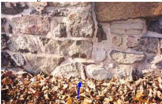
Vertical seam between units "A" and "B". Unit "A" water-table seen as shadow on "A" side of seam under plaque. Wooden beam aka "plate" just above door run length of unit "B" on south side.
