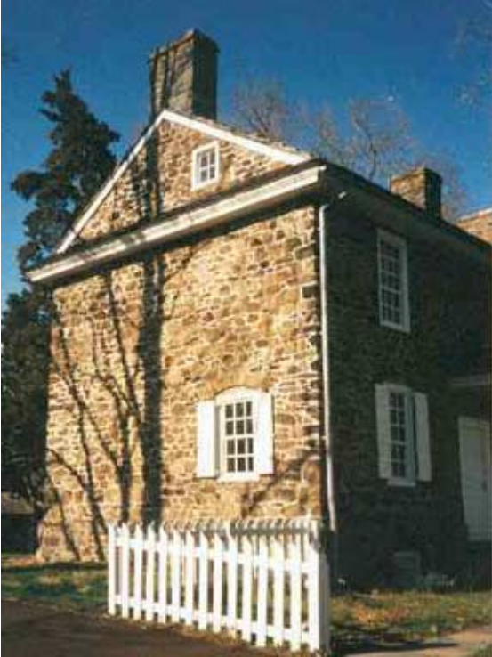
West end unit "A". Note Garret SW window, protruding ledge cornice. Once the east end of unit "A" looked like this, rotated 180° – it had a NE garret window. Note darker chimney stone.
