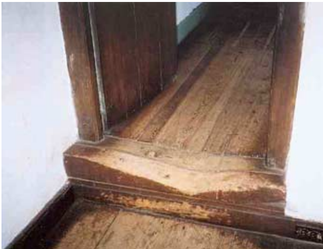
Door between units "A" and "B" is recessed in the wall, 4" to the west.
