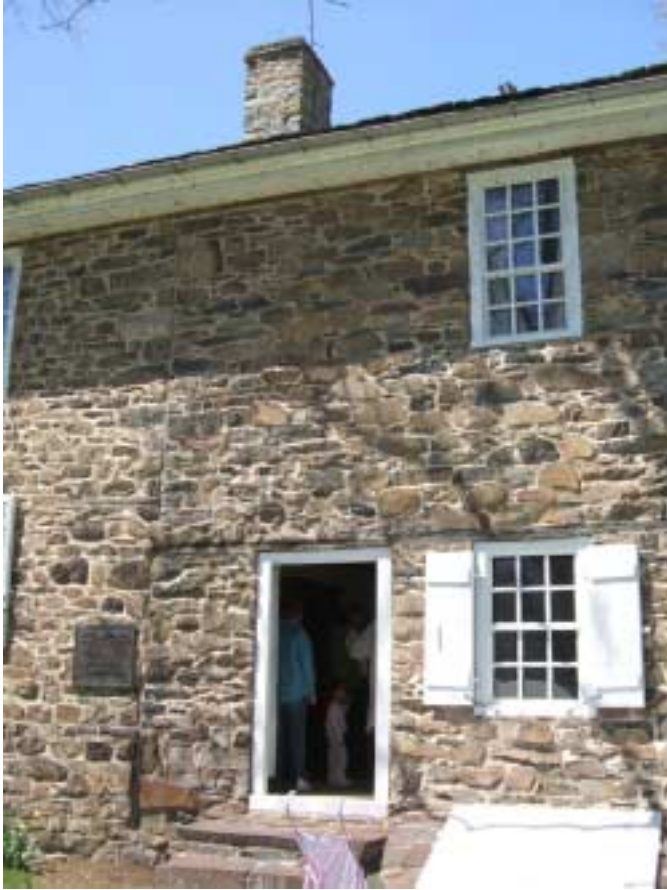
Vertical seam between units "A" and "B". Unit "A" water-table seen as shadow on "A" side of seam under plaque. Wooden beam aka "plate" just above door run length of unit "B" on south side.
