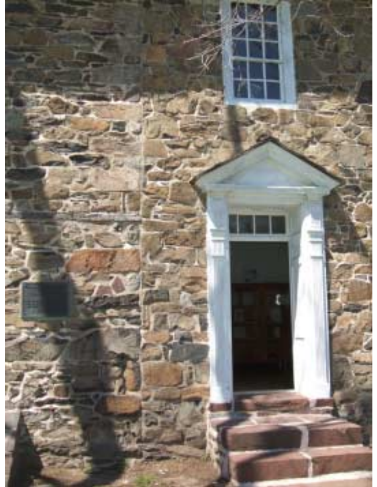
Vertical seam separating unit "B" from "C" on the right. Note large stone quoins forming SE but not SW corner of unit "B".
