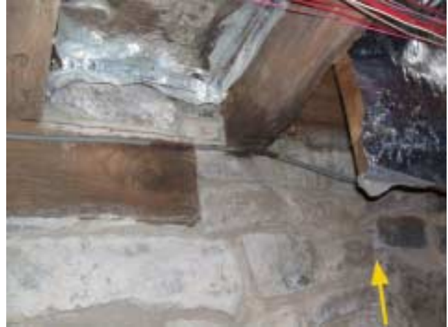
Summer beam embedded in west facing hearth extension (everything to left of yellow arrow) indicating floor was raised to new level when hearth extension added.
