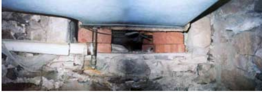
Opening in north wall "B0" to shed crawl space. HSR says wood sill [at base of opening] may date to an older structure. Brumbaugh says same for lintel (obscured by ductwork). West face Fireplace mass to right.
