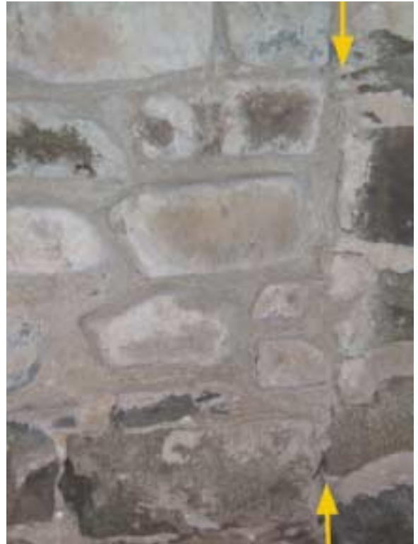
South edge of fireplace mass, showing vertical groove. Hearth extension is to the left.
