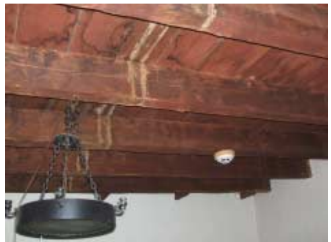
Unit "B", 2 nd floor shows East cornice supports protruding from the west wall, which once was the exterior wall of unit "A". The cornice protrusions are not supporting or connected to the unit "B" garret floor joists, that make up the ceiling.
